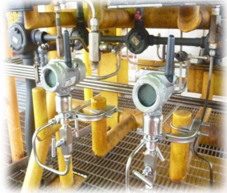
monitoring of Pressure in downspouts of wells. Caan A, Abkatun Pol Chuc
