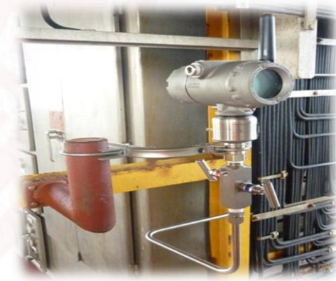
monitoring of the Pressure of the supply Hydraulic Console Baker, Chuc B, Abkatun Pol Chuc
